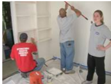
part of painting crew 4/26
