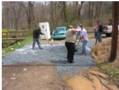
Driveway repair crew 4/19
