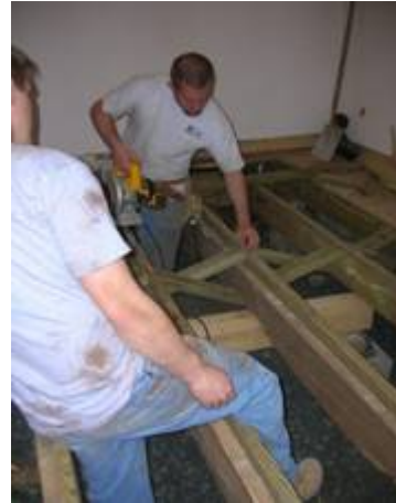
Floor repair crew 4/19
