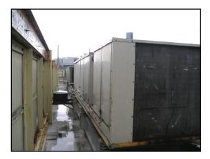
Pavilion Four and FH use No. 2 heating oil as their primary heat energy source. Two of the original "Nesbitt RMA" packaged, rooftop units on the RC roof were replaced in 2000/2001.
