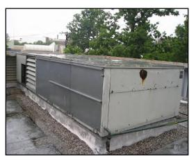
As discussed earlier, in the "Heating" section of this master plan, the most significant issue that stands out with regard to the existing East Campus building air conditioning systems is their age. The packaged, DX rooftop units are well beyond their "useful" mechanical life. The "expected median service life" of the packaged, DX rooftop units, is 15 years. The units predominantly used on the East Campus have been in service for 31 to 38 years.
