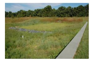
Similarly, the yard area around Darlington Hall has 3 micro-bioretention facilities plus an installation of pervious pavement on the south side. The micro-bioretention cells are carefully graded into the landscape close to the architecture and, in some cases, sculpted into narrow spaces between the building and the Thomas Run Road right-of-way. The permeable pavement is installed along a pedestrian pathway connecting the main building entrance with parking lot "C."
