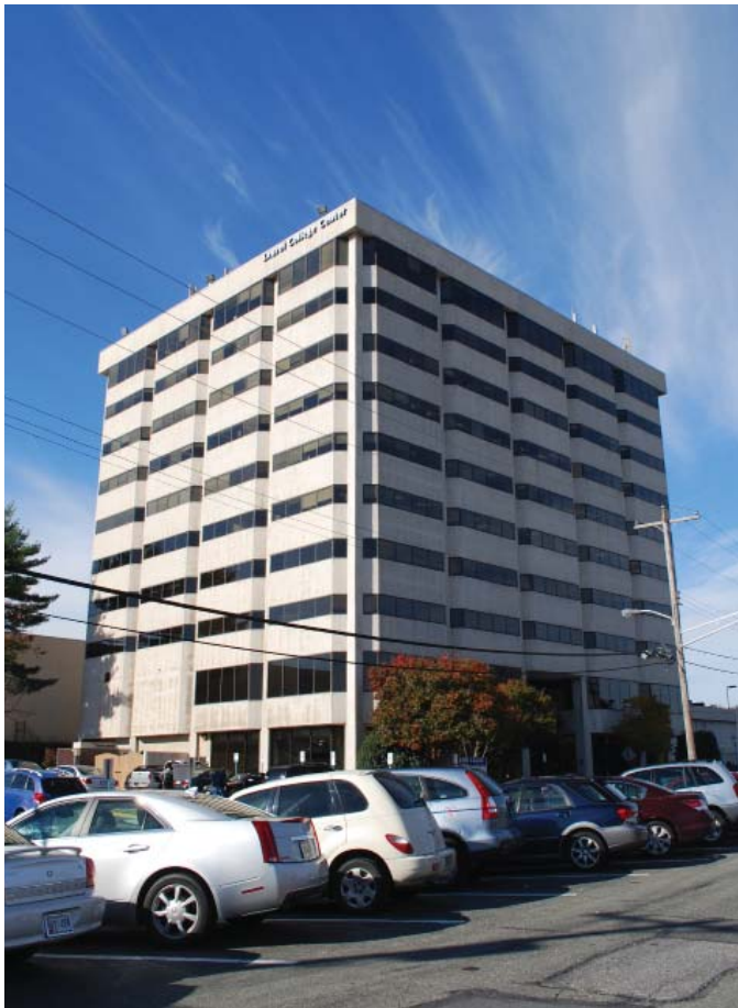
Laurel College Center - 312 Marshall Road, Laurel, Maryland
