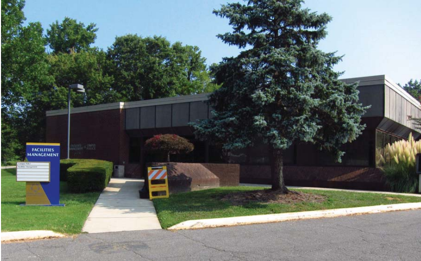
Brick-office portion of Facilities Management
