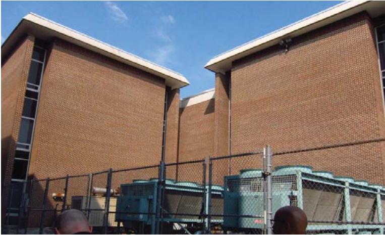
Lanham Hall and adjacent transformers Bridge connection between Lanham Hall and Largo Student Center
