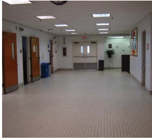
Excessively wide corridor on upper floor
