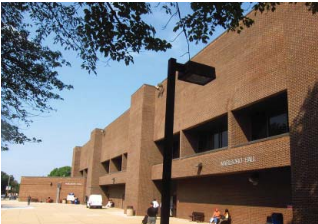
View of massive brick facade at east side
