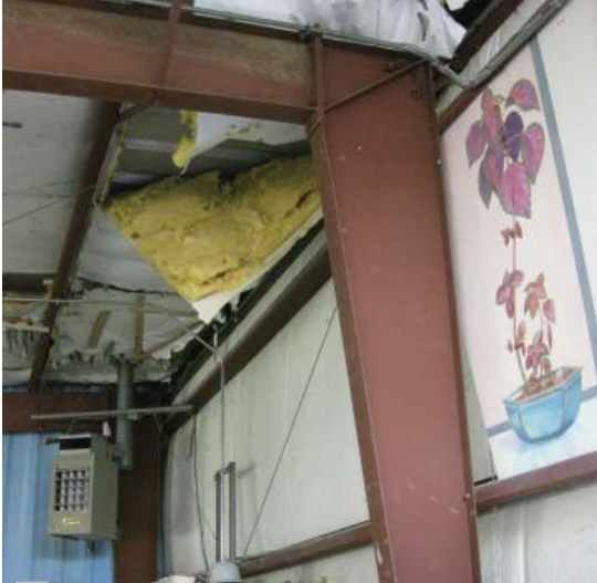
Ceramics Studio interior construction
