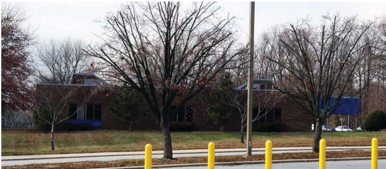
Exterior view from the outer ring road
