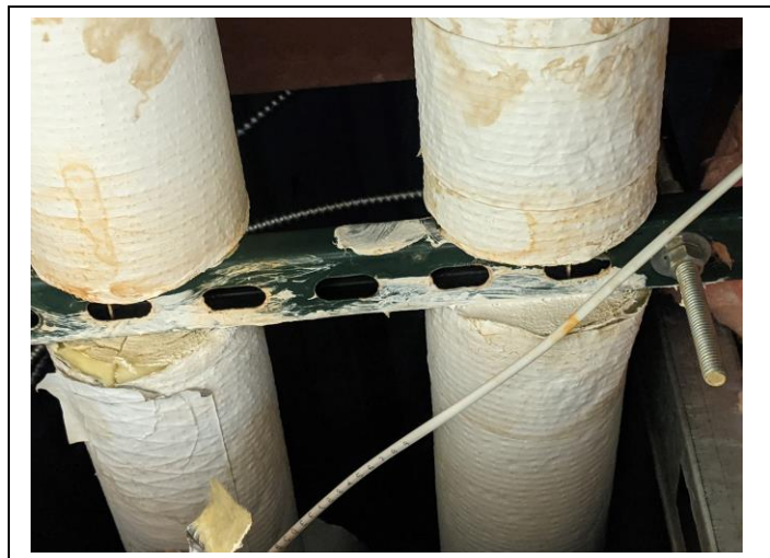
Photo #41 Material: White pipe seam sealant (on fiberglass) Sample location: AMA 1-27 No Asbestos Detected
