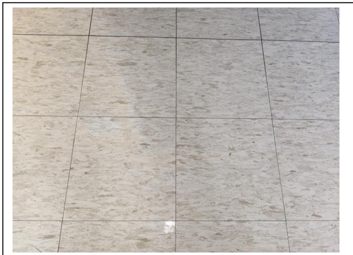
Photo #5 Material: 12"x12" Tan mottled floor tile Sample location: AMA 2-48 (2% Chrysotile)
