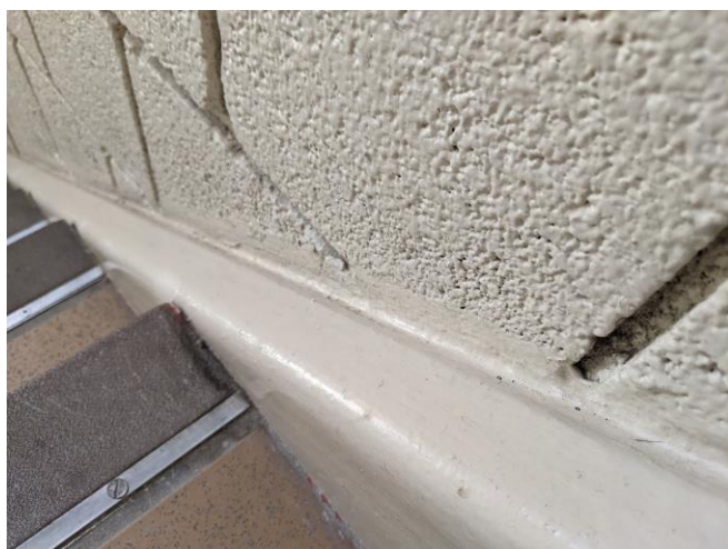
Photo #47 Material: White wall caulk Sample location: AMA S-1 No Asbestos Detected
