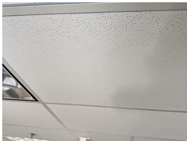
Photo #29 Material: 2'x4' Multi-size pinholed ceiling tile Sample location: AMA 1-01 No Asbestos Detected
