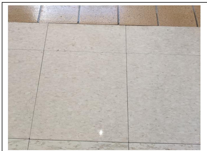
Photo #8 Material: 12"x12" Beige mottled floor tile Sample location: AMA S-1 Adhered to asbestos-containing black floor tile mastic
