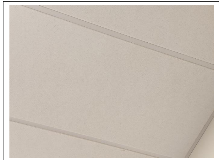
Photo #28 Material: 2'x4' Textured/pinholed ceiling tile Sample location: AMA 1-01 No Asbestos Detected
