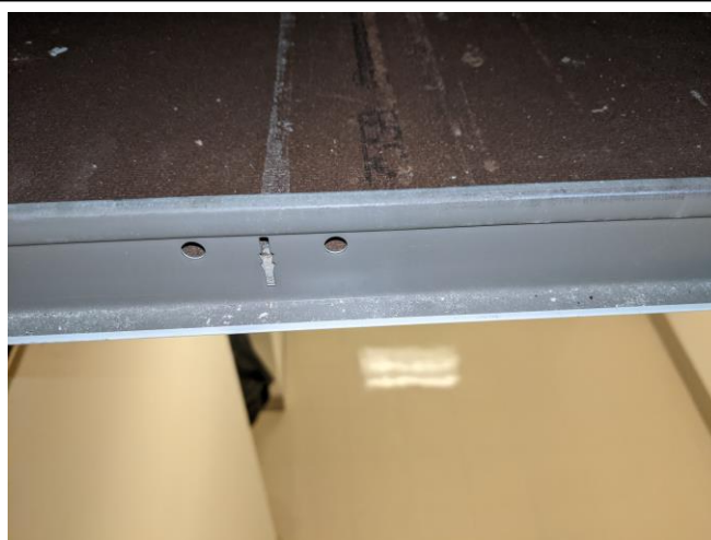
Photo #32 Material: 2'x4' Fissured/pinholed ceiling tile (brown backing) Sample location: AMA 1-27 No Asbestos Detected
