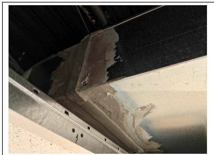
Photo #42 Material: Gray metal duct seam sealant Sample location: AMA 2-48 No Asbestos Detected
