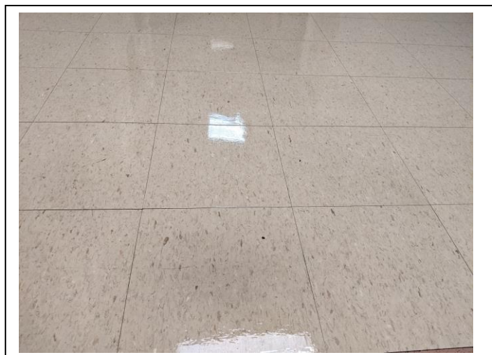
Photo #7 Material: 12"x12" Tan with brown specks floor tile Sample location: AMA 1-19 Adhered to asbestos-containing black floor tile mastic
