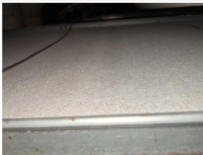
Photo #30 Material: 2'x4' Cratered/pinholed ceiling tile (base backing) Sample location: AMA 2-48 No Asbestos Detected
